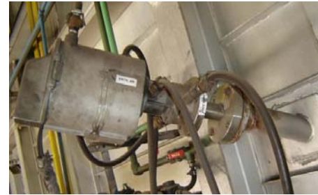
Furnace Camera with F31 Flange Mount
