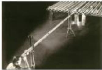
Anti-aircraft gun plant, inspection of rifling & interior finish, 1942
